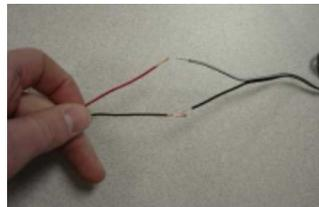
Step 2: Now take the red power cable lead and twist it together with the black & white lead from the power pigtail. Now take the black lead from the power cable and twist it together with the all black lead from the pigtail. Use the gray wire nuts provided with your system and twist them onto the wires until they are firmly secured.
